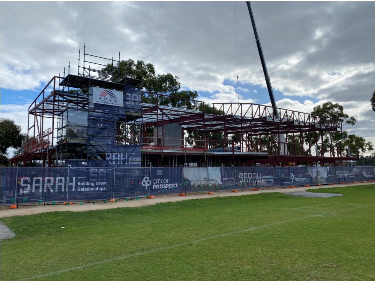
IMAGE 3: SUPERSTRUCTURE FACING EAST WITH LIFT SHAFT VISIBLE & TEMPORARY GRAVEL WALKWAY
