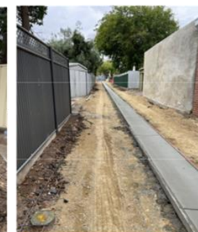
James Street and Redin Street kerb and gutter construction
